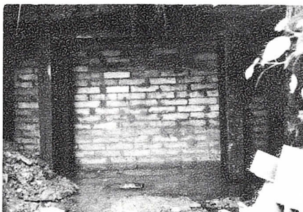
Seal in place. Eight open entryways were sealed keeping surface water and children out of the old mines.
