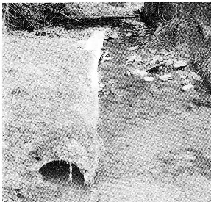
A "wildcat" sewer discharges raw sewage into Bushy Run near Manor. This and many other open discharges will be collected and treated in the new system.
