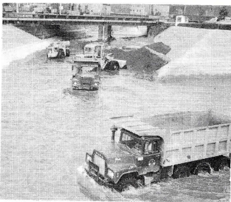
Sediment removal at the mouth of Thompson Run during 1972 cleaning.
