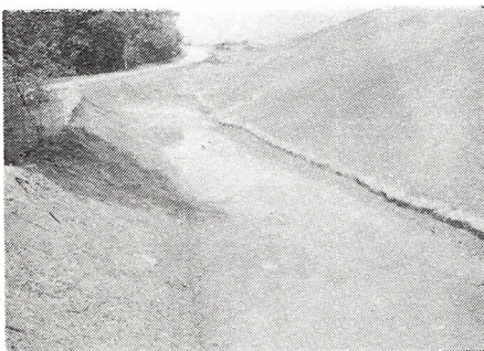
A large detention pond serving the East Suburban Hospital in Monroeville absorbs storm runoff, and safely discharges the water to nearby streams when the storm has passed.
