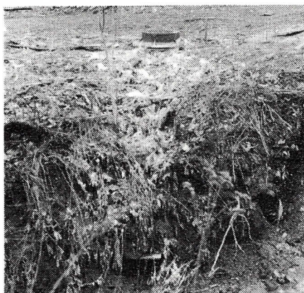
Raw sewage shown here seeps from a manhole into Thompson Run when flow rates are high.
