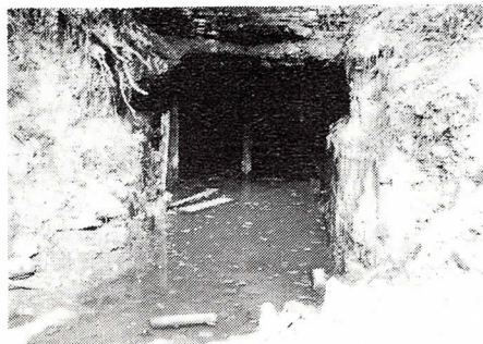
Surface water enters the tunnel system of the Irwin Syncline through an old pit mouth. DER has since sealed this entrance.
