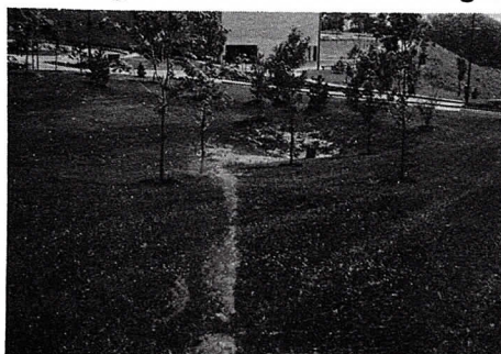
Detention ponds, such as this one in operation collecting runoff from the parking lots of the East Suburban Hospital in Monroeville, can protect downstream areas, and fit into the landscaping, too.
