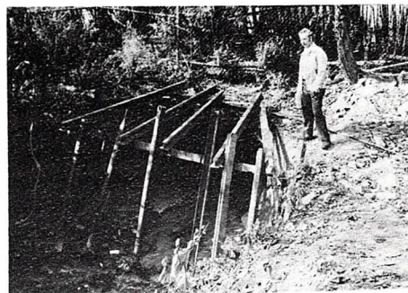
Jeff Loser, SCS District Conservationist, looks at the six-foot diameter culvert just above the Turtle Creek football field. This pipe will determine, to a large extent, the maximum sizing of upstream pipes.
