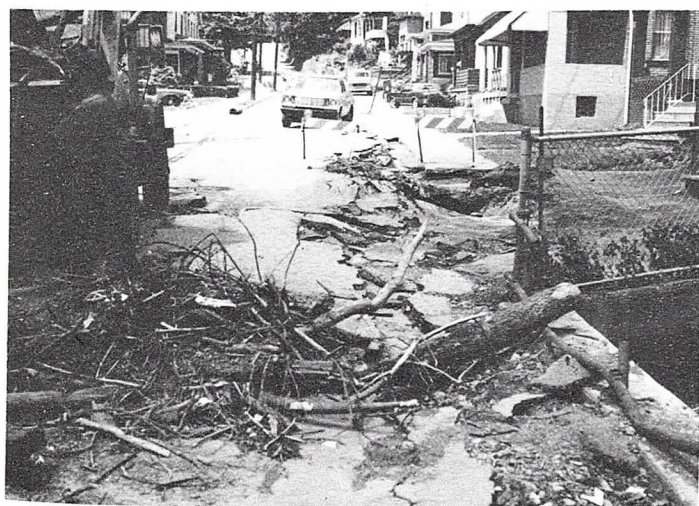
Heavy damages wrought by the June 9th flood were inflicted on Sawmill Run retaining walls, State Route 130 and adjacent properties in the Borough of Turtle Creek. At times, water was 2 to 3 feet deep on the roadway at this location.
