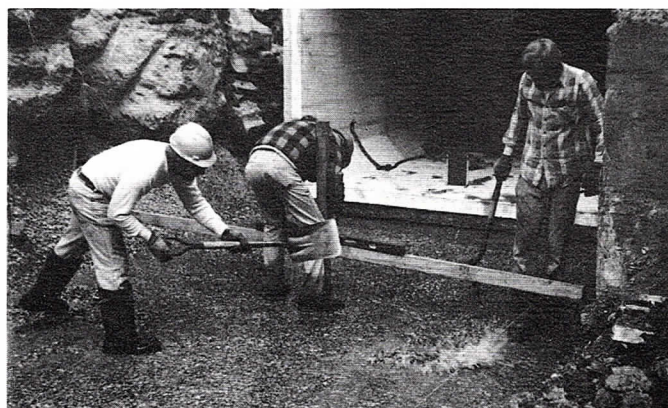
Bedding of slag is leveled to receive another six-foot section of culvert. The second phase of the project is expected to start during the Summer of 1982.
