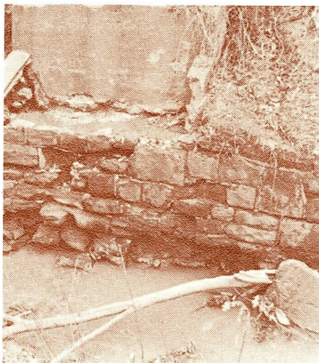
Undercutting of wall requires concrete footer.
