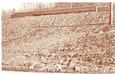
Unseeded construction site shows quick way to get sheet erosion into Commonwealth streams: leave catchbasins unprotected. Bales of hay around this drop inlet would adequately keep sediments from entering the storm sewer system.
